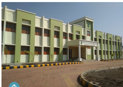
School Building constructed under Vardhman School Development Program - Government Excellence Higher Secondary School, Obedullaganj, Mandideep, MP
