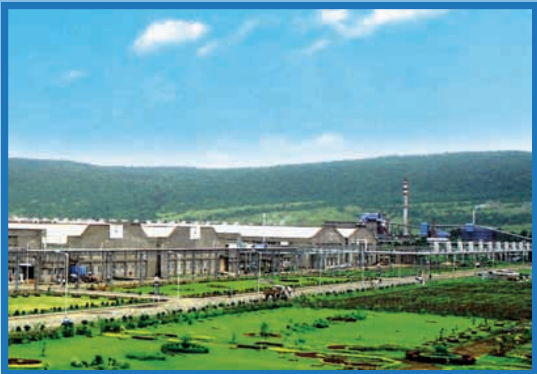
A panoramic view of Vardhman Fabrics, Budhni, a unit of the Company.
