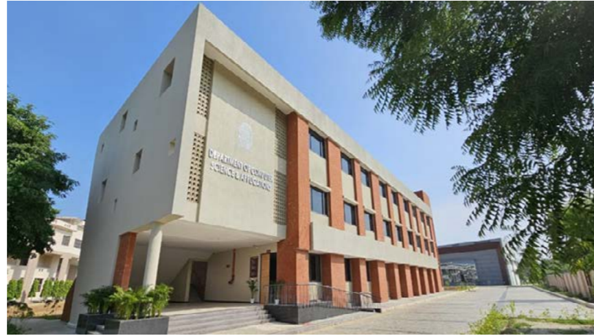
Construction of new block – "Dept. of Computer Science and Applications" at SACCM, Ludhiana
