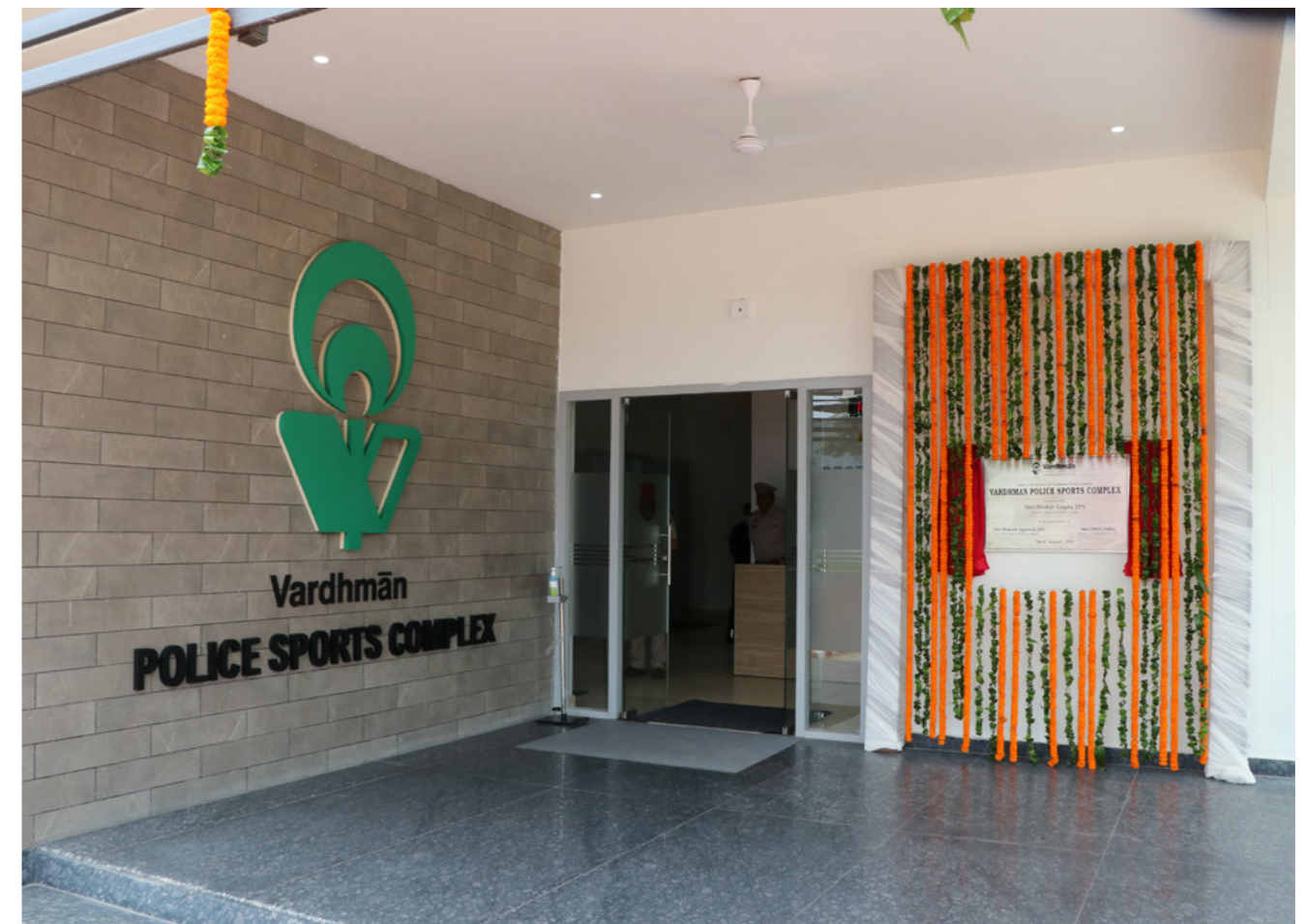
Constructed Indoor Badminton Hall and Gymnasium at Police DAV School, Civil Lines Ludhiana
