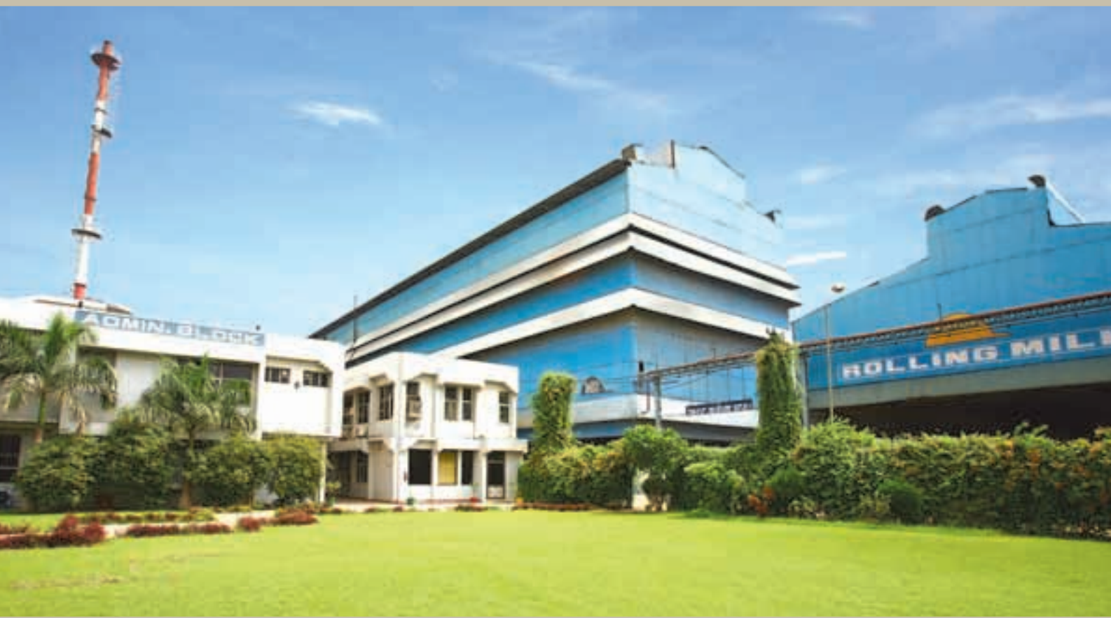
A scenic view of the Company's unit, Vardhman Special Steels Limited Unit-I, Ludhiana
