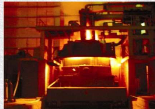
Two Ladle Refining Furnace
