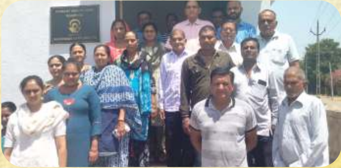
Primary Health Care Centre constructed at Ranipura Village, Jhagadia, Gujarat
