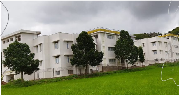
Constructed Hostel for Tribal Girls at Kechla, Odisha
