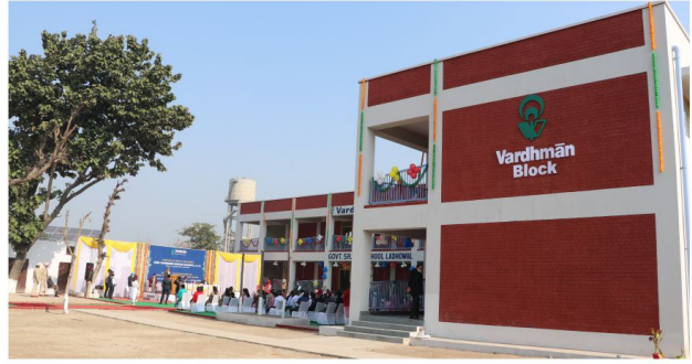
Vardhman Block at Government Senior Secondary School, Ladhawal, Ludhiana Total Students Benefitted : 819
