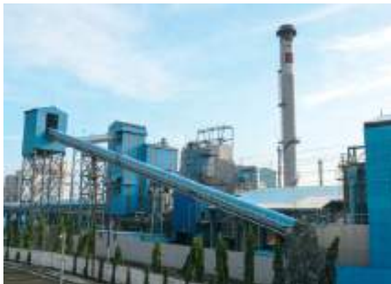
40 TPH Boiler, Baddi
