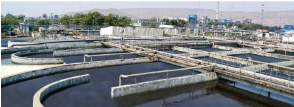
ETP at Vardhman Fabrics, Budhni
