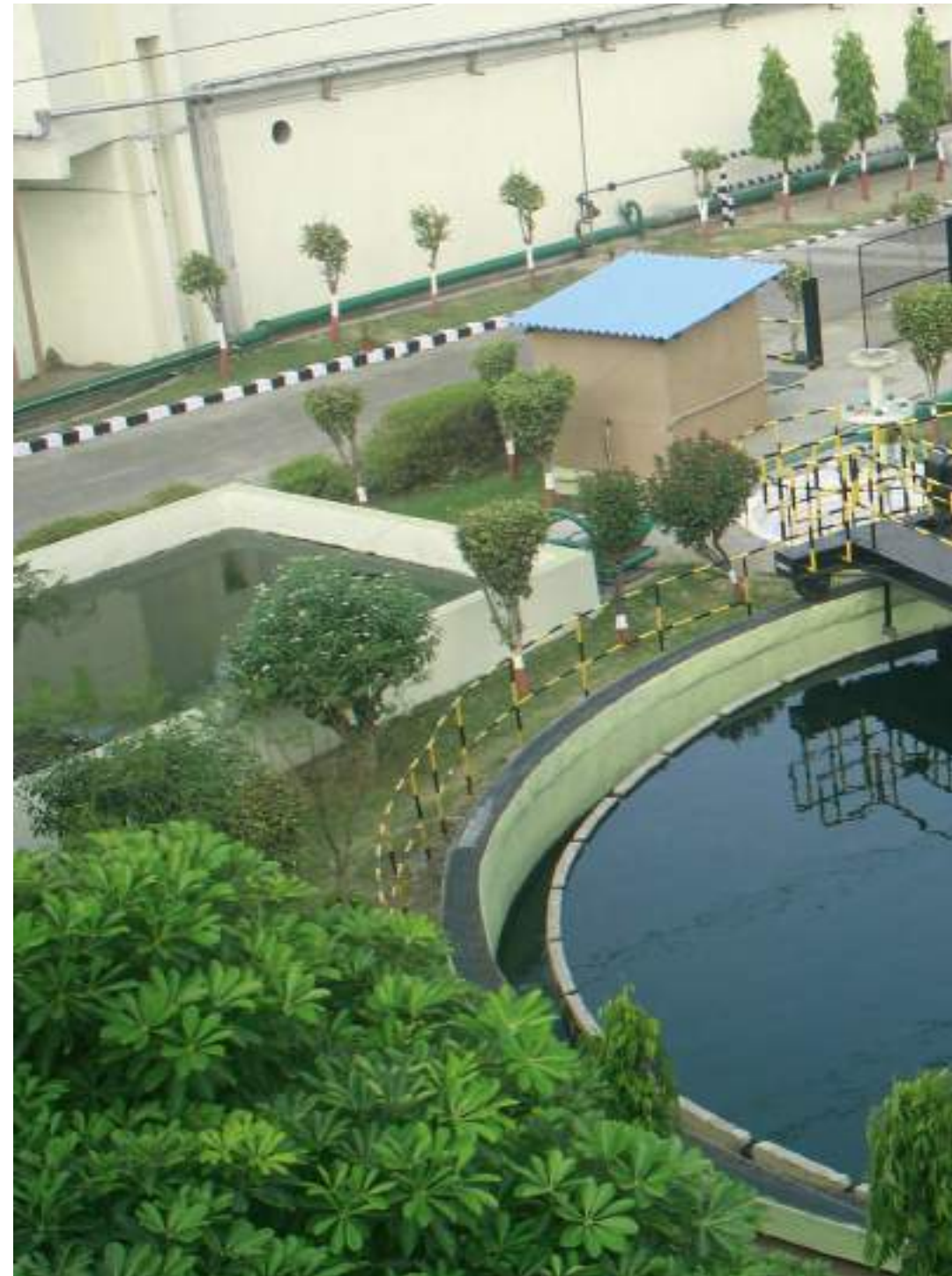
Effluent Treatment Plant, Ludhiana
