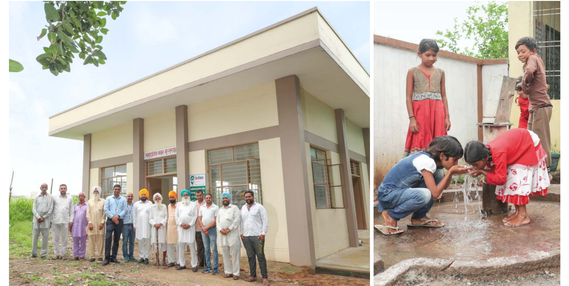
Community members pose with pride in front of the Community Hall constructed by Vardhman, Baddi
