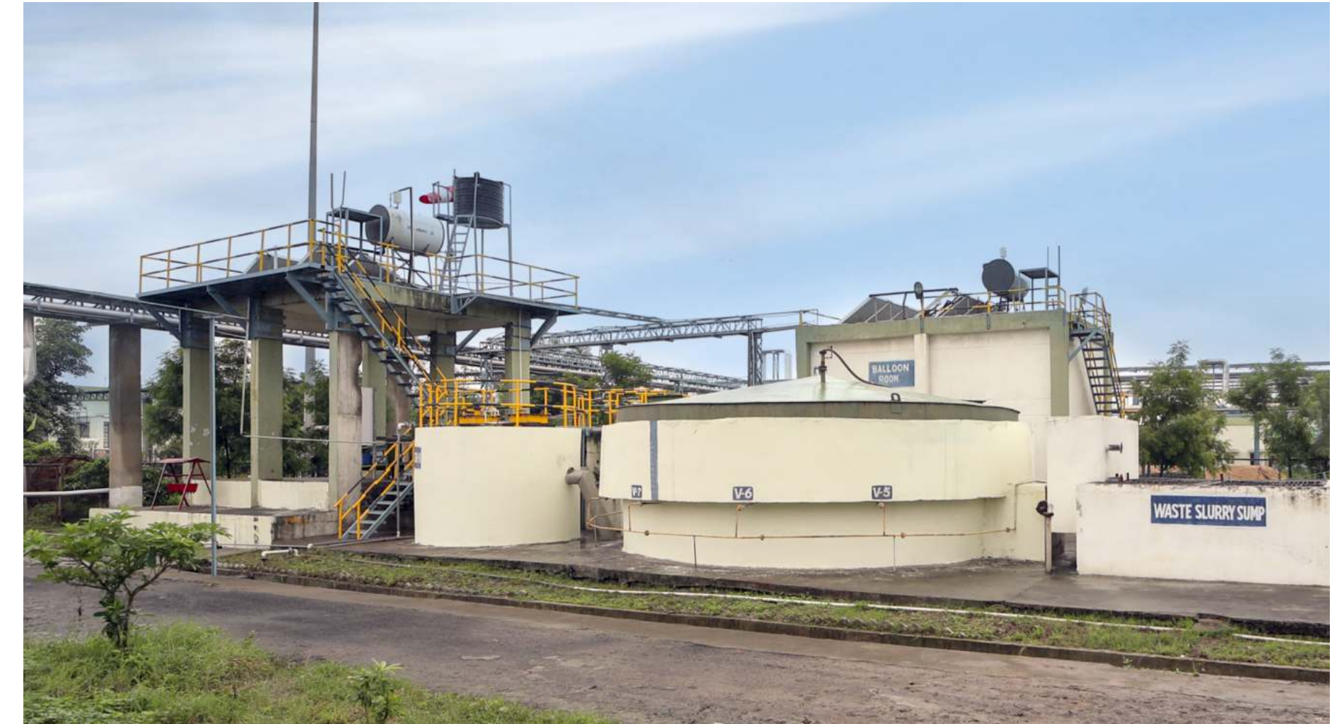
Biogas Plant - Vardhman Fabrics, Budhni
