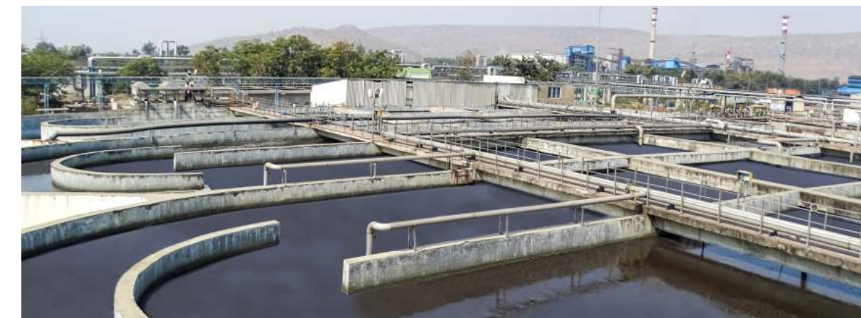
ETP at Vardhman Fabrics, Budhni
