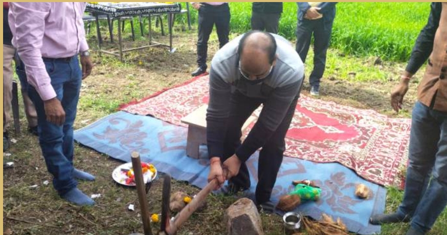
Bhumi Poojan for the Construction of Activity Hall at Govt. Middle School, Khandabad, MP.
